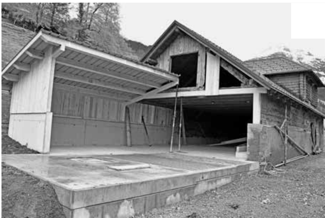
Anbau Alphütte Bettenebnet
